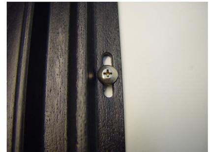
**NOTE:** Pre-drilling holes for the screws in the glides or trailer are not required if the trailer deck is wood. The screws supplied with this kit are not meant to be used in steel or aluminum, but can be if an 11/64" drill bit is used first to drill a pilot hole. Caution should be used in areas where marker lights and wires have been installed under the trailer deck when installing all fastener.
